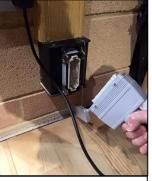
A multi-pin connector allows the console to be connected via a single socket. This speeds up set-up whilst allowing the console to be stored when not in use.
